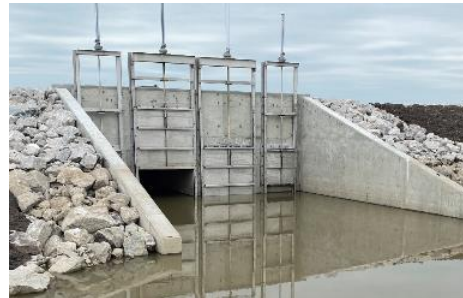
Clarence Cannon Water Control Structure MVS
