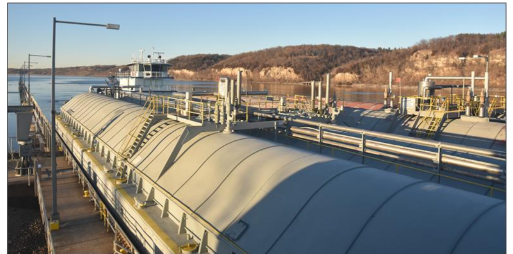
Motor Vessel Richard E. Waugh, Lock and Dam 10
